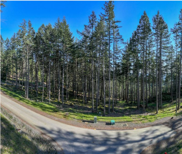
The entrance road as built, spring 2025. Photography: David Strongman.
